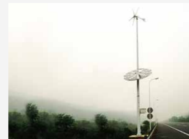
Sky Driven system power 7pc 85W LED street light – suburb Guangzhou 2011
