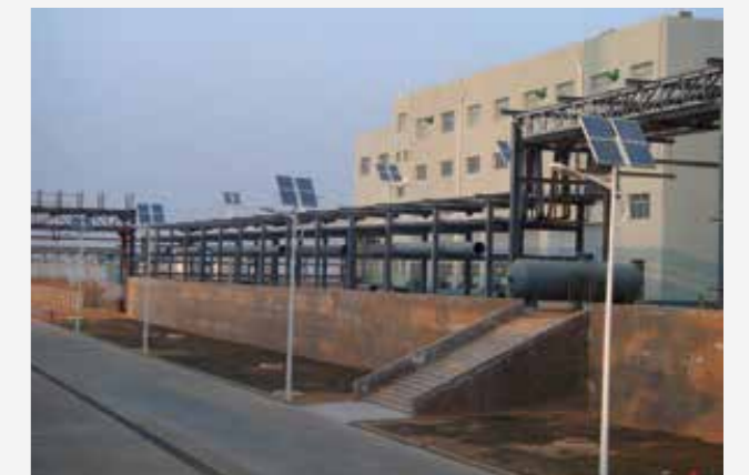
45W LED solar lighting for factory plant - Guangzhou China 2010
