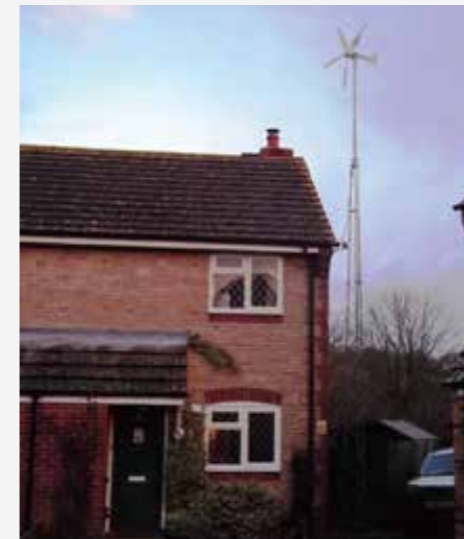
DM-1000 grid-tie system with lattice tower - Liverpool UK- 2009
