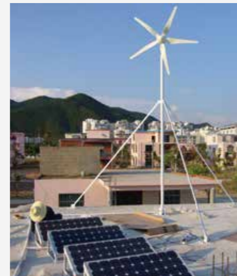
1KW wind solar hybrid off-grid power system for residential - Hainan Island China - 2007
