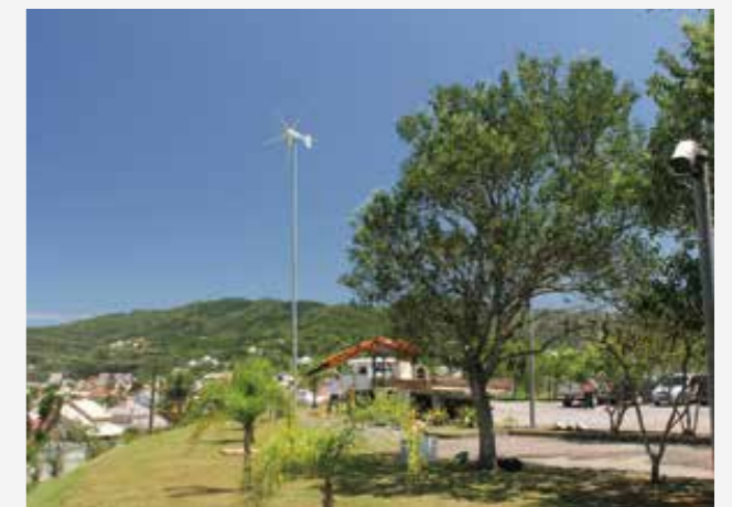
DM-3000 grid-tie system with 13.4m hydraulic tower installation - Florianopolis Brazil 2010
