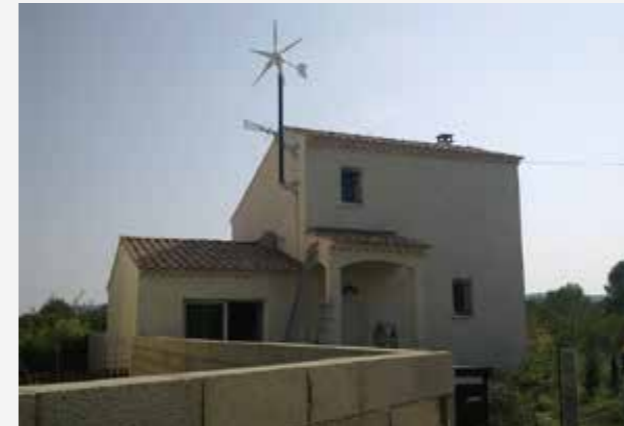
DM-1000 grid-tie system with wall fixation installation - Lyon France - 2011
